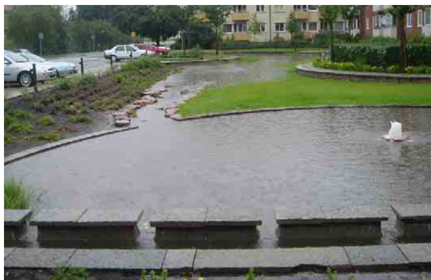
Figure 48. Controlled flooding of the “double pond” during extreme wet weather conditions
