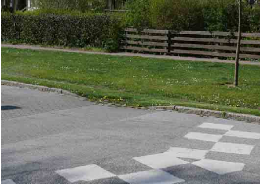
Figure 27. Close up of one of the concave traffic bumps in the Vanåsgatan
