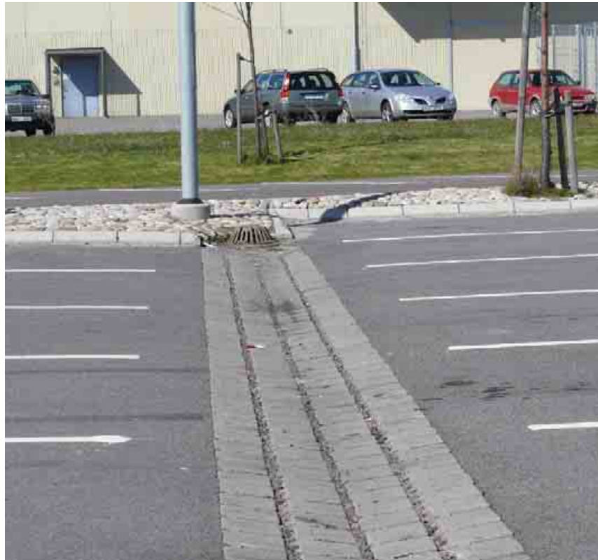
Figure 29. Runoff from a parking areas is diverted to stone fillings
