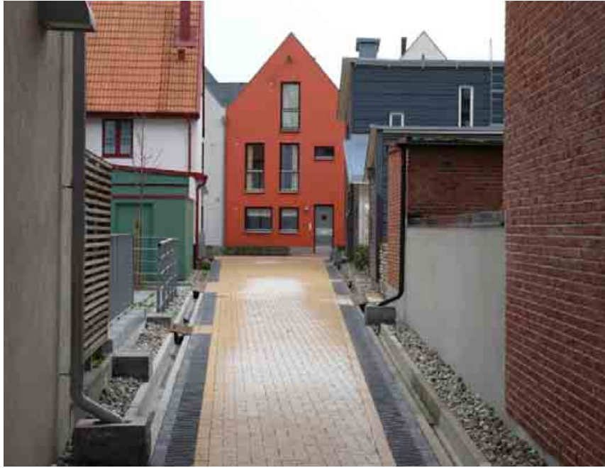
Figure 63. Drainage canals in the housing exhibition area Bo 01
