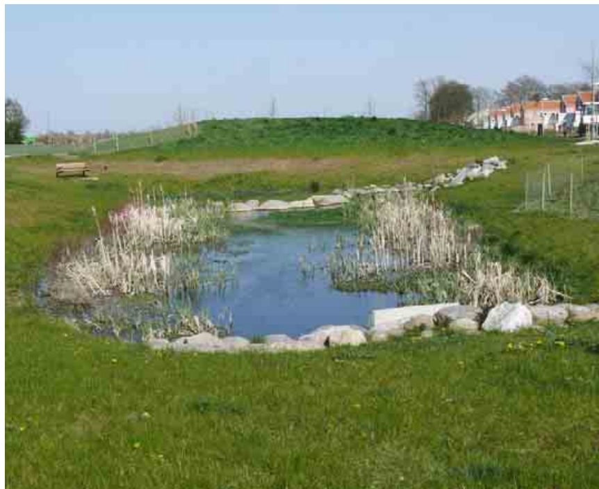
Figure 91. The detention pond in the upstream end of the Växthusparken Eco-Corridor
