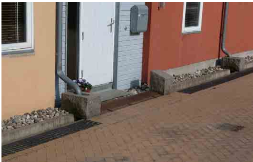
Figure 64. Detail of a drainage canal in the housing exhibition area Bo 01
