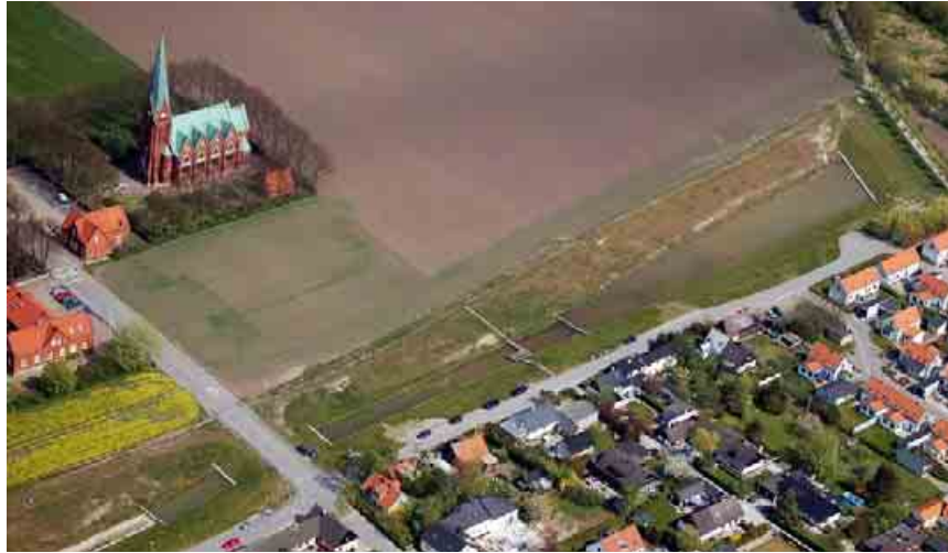
Figure 85. Aerial view of the upper part of the Vintriediket Drainage Corridor
