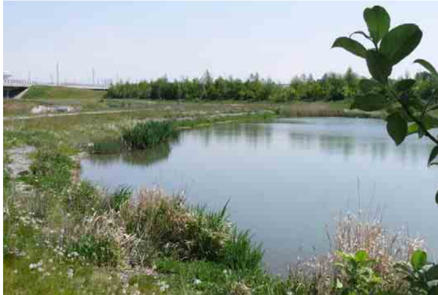
Figure 82. View of the filter bank in the eastern pond at the Gottorpsvägen
