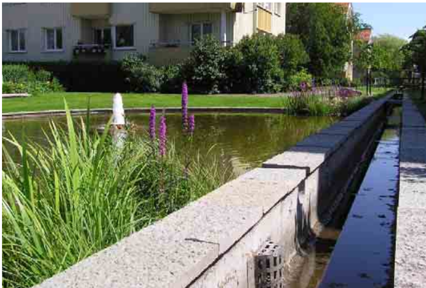
Figure 45. Water is led from the drainage canal to the upper pond
