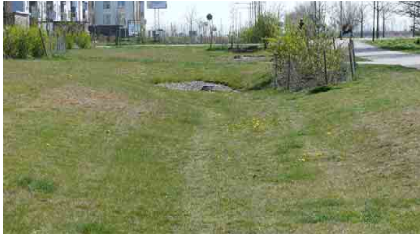
Figure 88. Onsite detention in a swale within the settlement of Annestad
