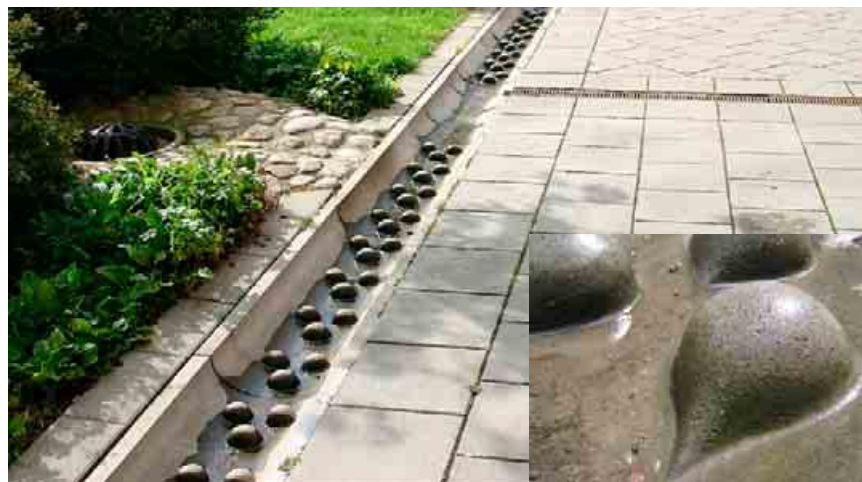
Figure 44. "Water drop" gutter diverting water from the downpipes of the apartment blocks to the concrete drainage canal
