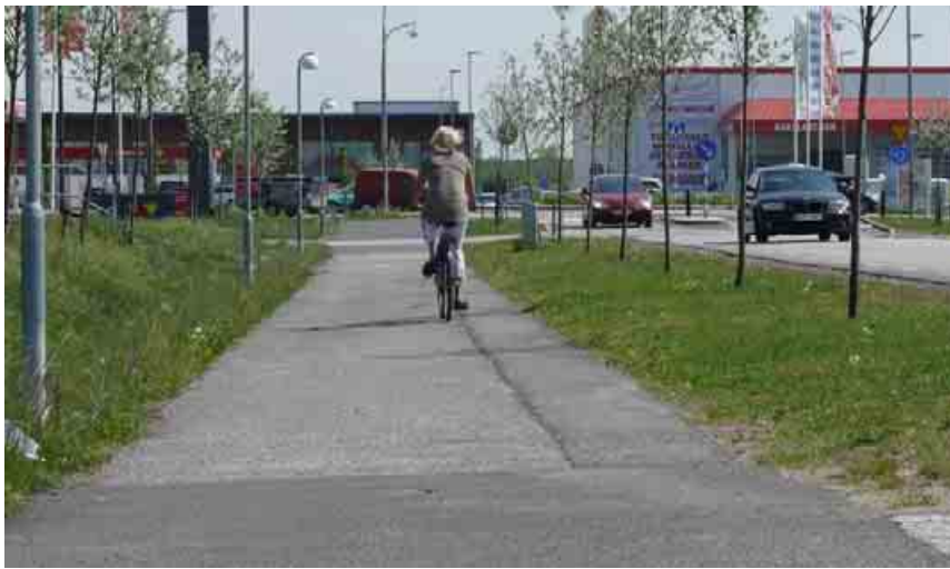
Figure 30. Depression storages along one of the streets in the Svågertorp Business Centre
