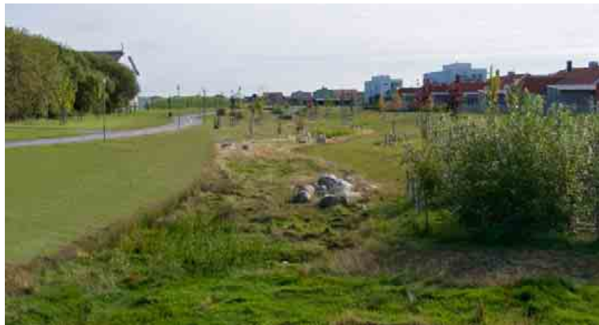
Figure 76. The downstream end of the eastern part of the Fjärilsparken Eco-Corridor is completed.
