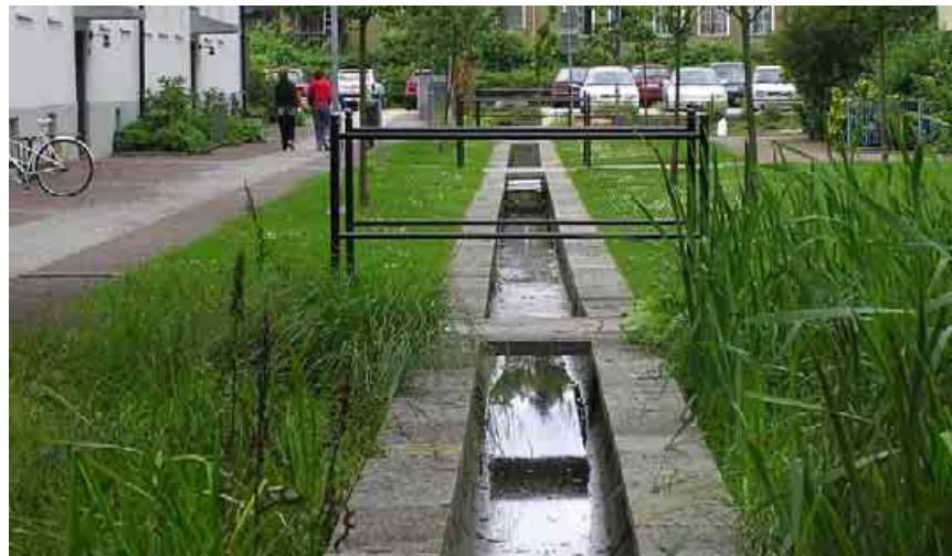
Figure 43. Mini-wetland at the concrete canal in the upper section of the Central Drainage Corridor
