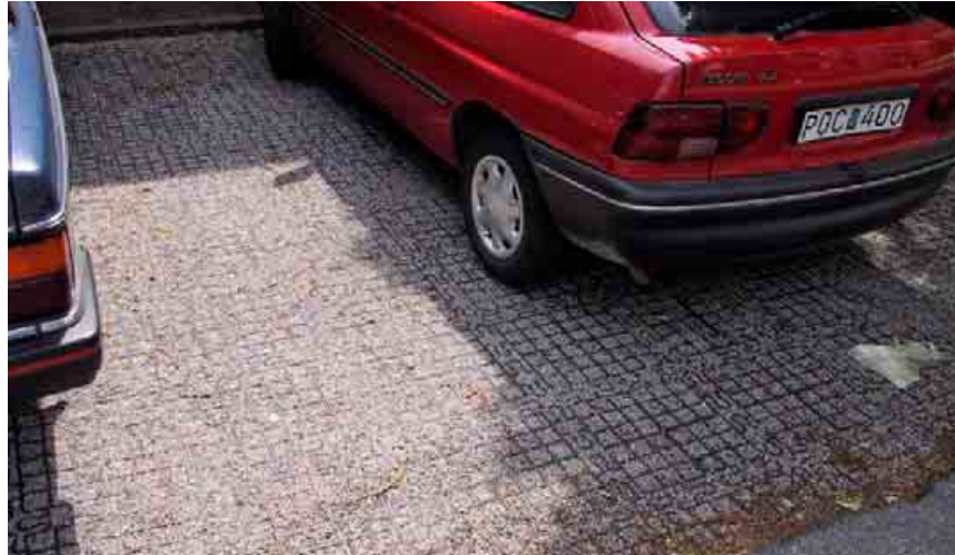
Figure 56. Permeable parking built up of coarse gravel and stabilized with a grid of hard polyethylene
