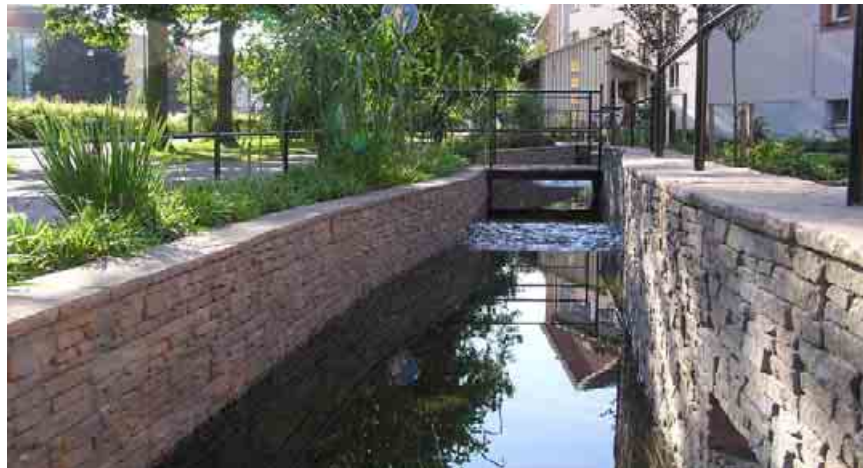
Figure 54. The canal section in the lower part of the Lönngatan Drainage Corridor
