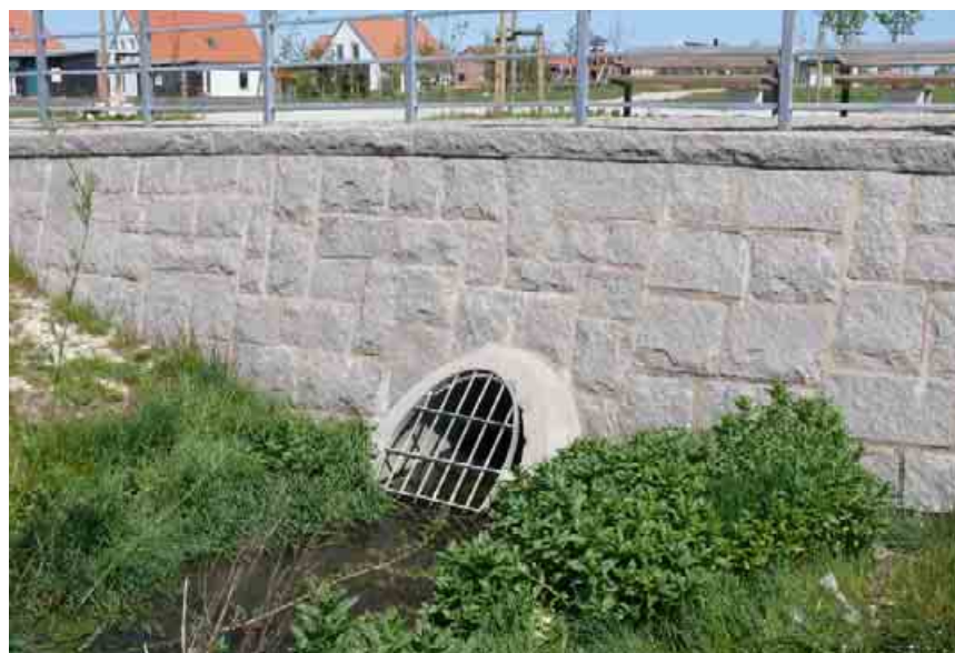
Figure 93. Water is entering the upper watercourse through a stone wall
