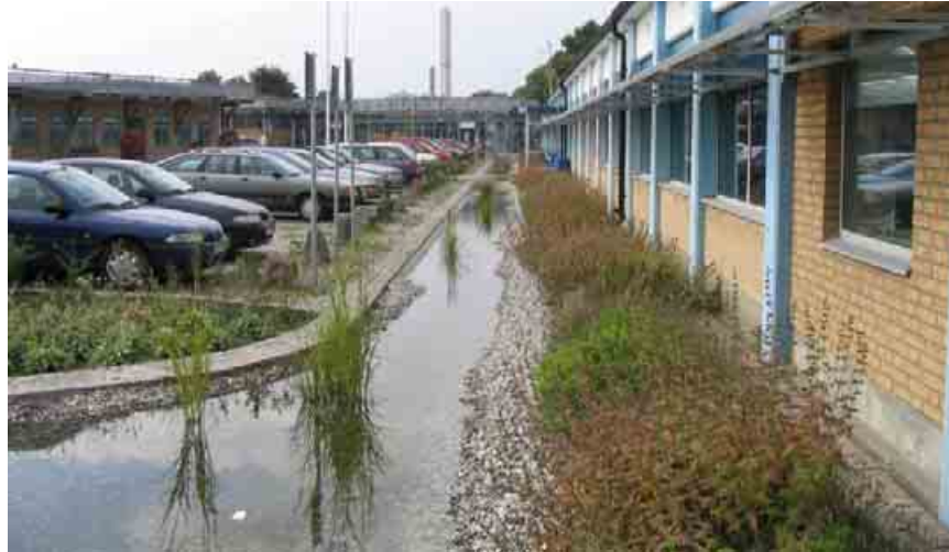
Figure 42. All excess water from the green roofs is collected in an open drainage canal
