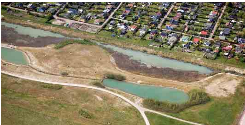
Figure 78. Aerial view of the detention ponds in the Elinelund Recreation Area
