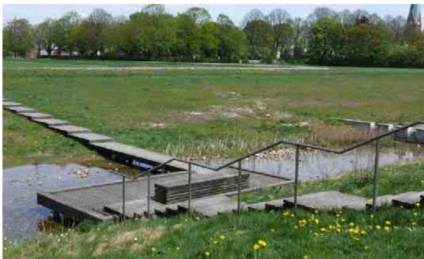
Figure 87. Wooden platforms in the ponds of the Vintriediket Drainage Corridor
