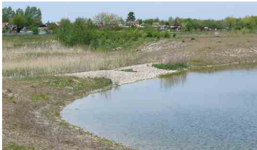
Figure 80. The filter wall in the second pond in the Elinelund Recreation Area
