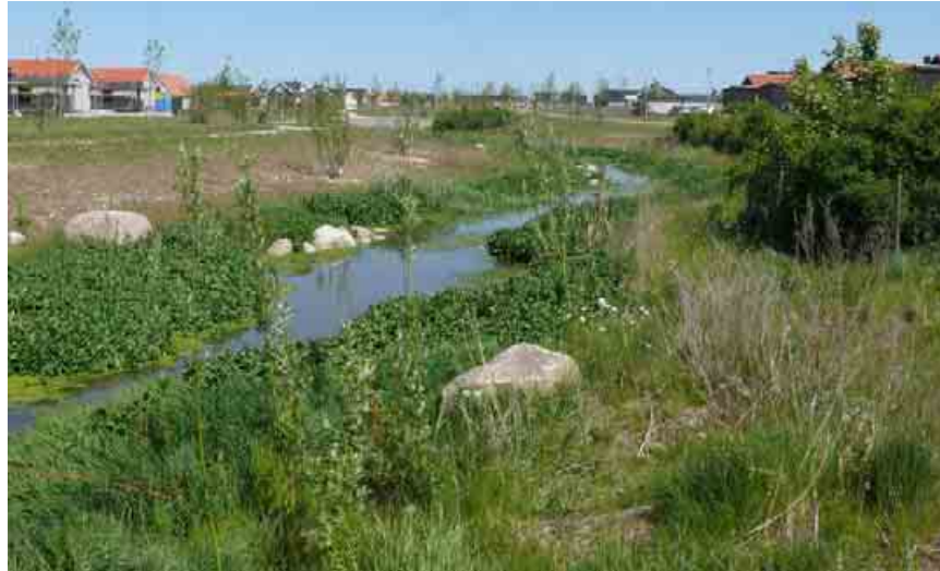
Figure 94. The watercourse is meandering through the local park in the upper part of the Tygelsjö Eco-Corridor
