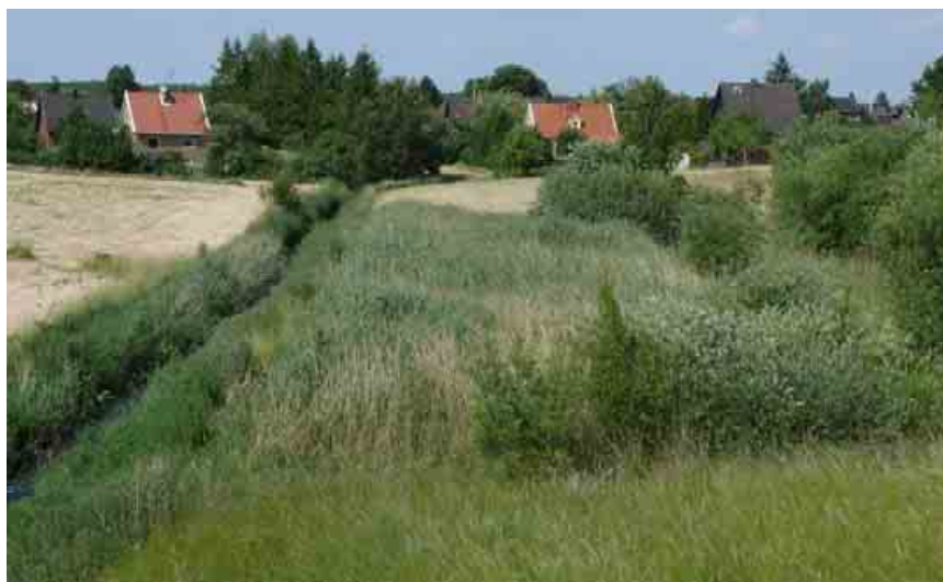
Figure 15. Overview of the root-zone facility at the downstream end of the Sallerupsvägen Drainage Corridor
