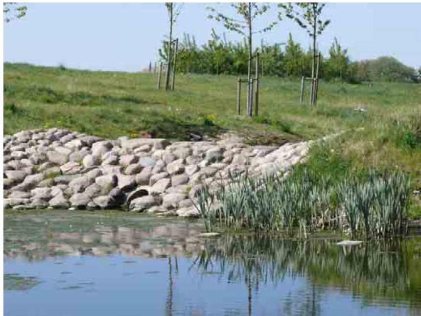
Figure 98. The outlet structure in the big pond in the Tygelsjö Eco-Corridor
