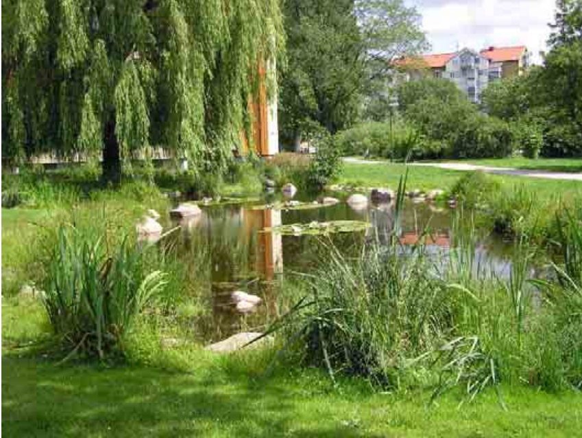
Figure 59. A local detention pond located close to the public park in the settlement of Augustenborg
