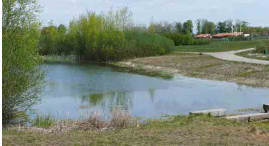
Figure 79. View of the first pond and the outlet structure
