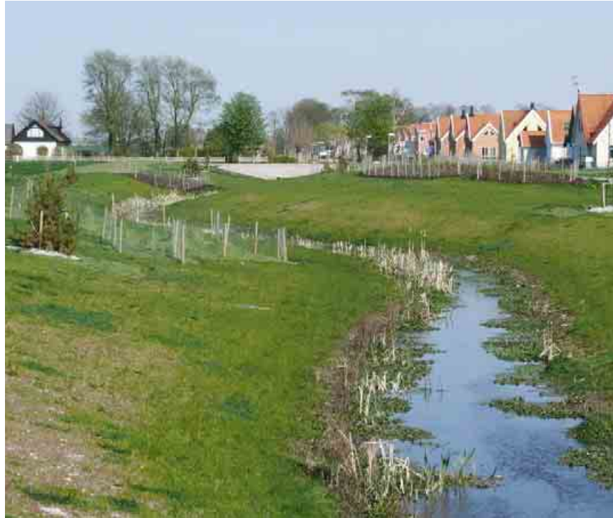
Figure 90. View of the meandering watercourse in the Växthusparken Eco-Corridor
