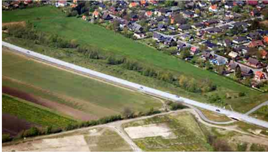
Figure 13. Aerial view of the Sallerupsvägen Drainage Corridor.
