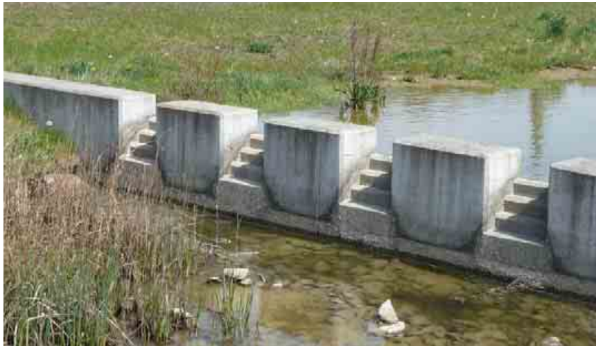
Figure 86. Overflow openings in the concrete wall between the ponds
