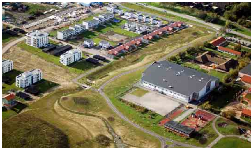
Figure 77. An aerial view of the downstream end of the eastern part of the Fjärilsparken Eco-Corridor.
