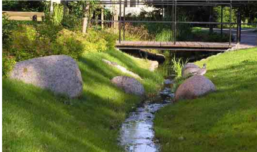
Figure 53. The swale in the lower part of the Lönngatan Drainage Corridor
