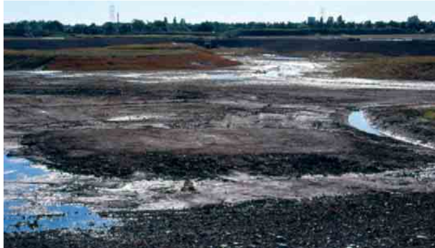
Figure 6. Excavation work during the construction of the Toftanäs Wetland Park
