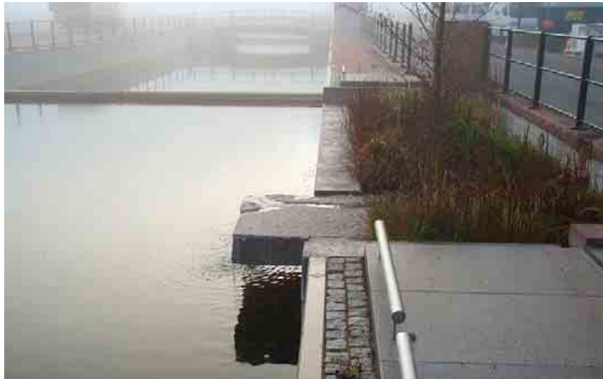
Figure 66. Collection chamber for stormwater located at the saltwater canal.
