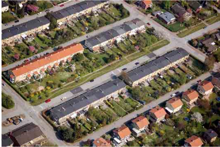
Figure 25. Aerial view of one section of the Vanåsgatan Swale
