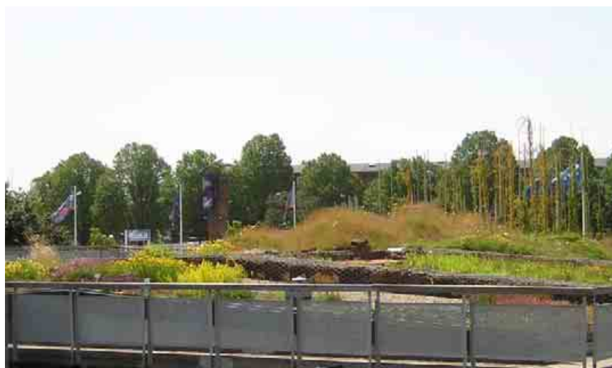
Figure 36. Overview of one section of the Augustenborg Botanical Roof Garden
