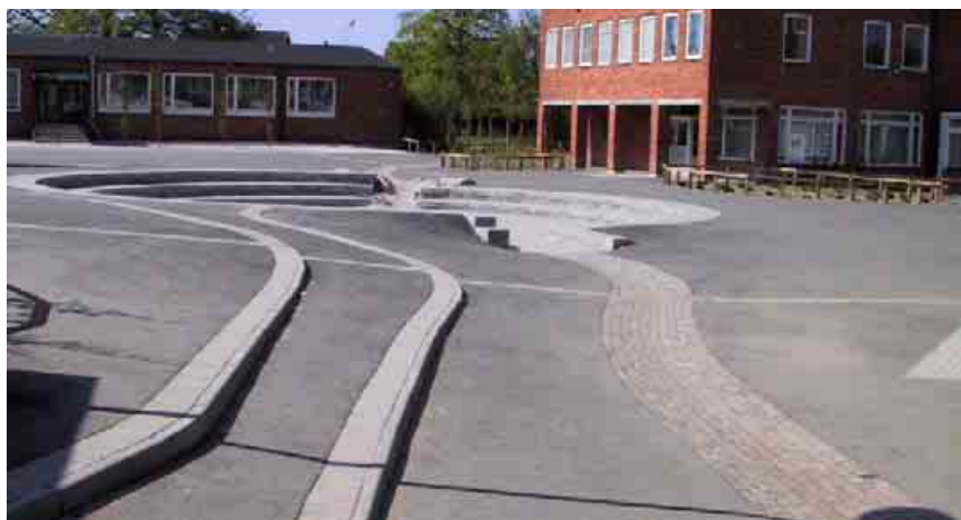
Figure 58. Open detention in an "amphitheatre" in the schoolyard in the settlement of Augustenborg
