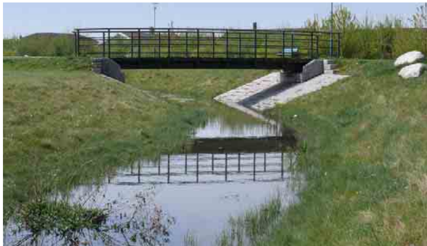
Figure 89. Detention in a vegetated canal in the settlement of Annestad
